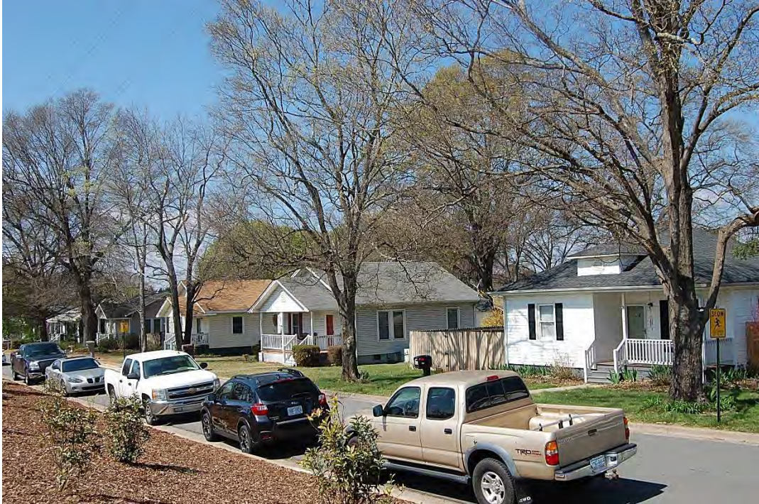
Belmont Fabric Company-South Fork Manufacturing Company Mill Village, 100 Block of Live Oak Avenue, Looking Northwest From Modern Berm.
