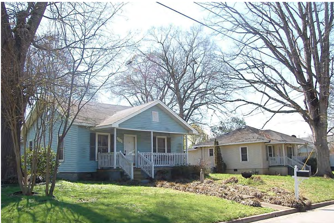
Belmont Fabric Company-South Fork Manufacturing Company Mill Village, 103-105 Rankin Street, Looking Southwest.
