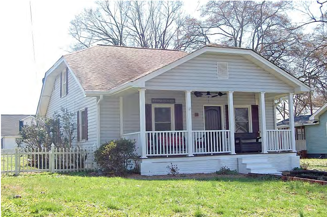
Belmont Fabric Company-South Fork Manufacturing Company Mill Village, Supervisor's House, 101 Rankin Street, Looking South.
