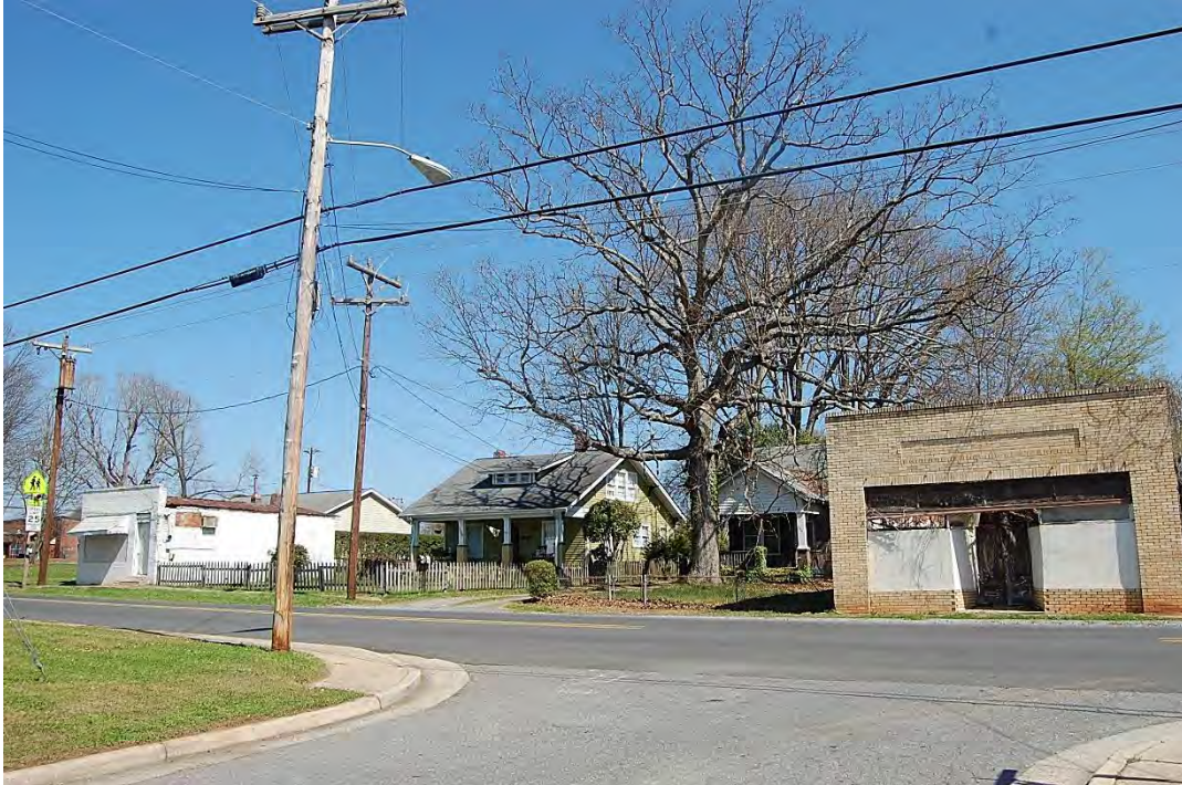
Stowe Spinning Company Mill Village, 1920, Woodlawn Street at Belmont Avenue, Belmont, Looking West.
