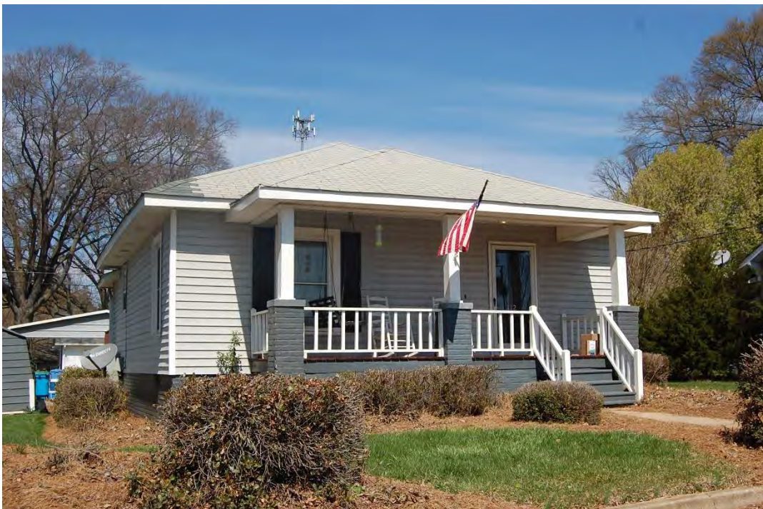
Belmont Fabric Company-South Fork Manufacturing Company Mill Village, 116 Live Oak Avenue, Looking North.
