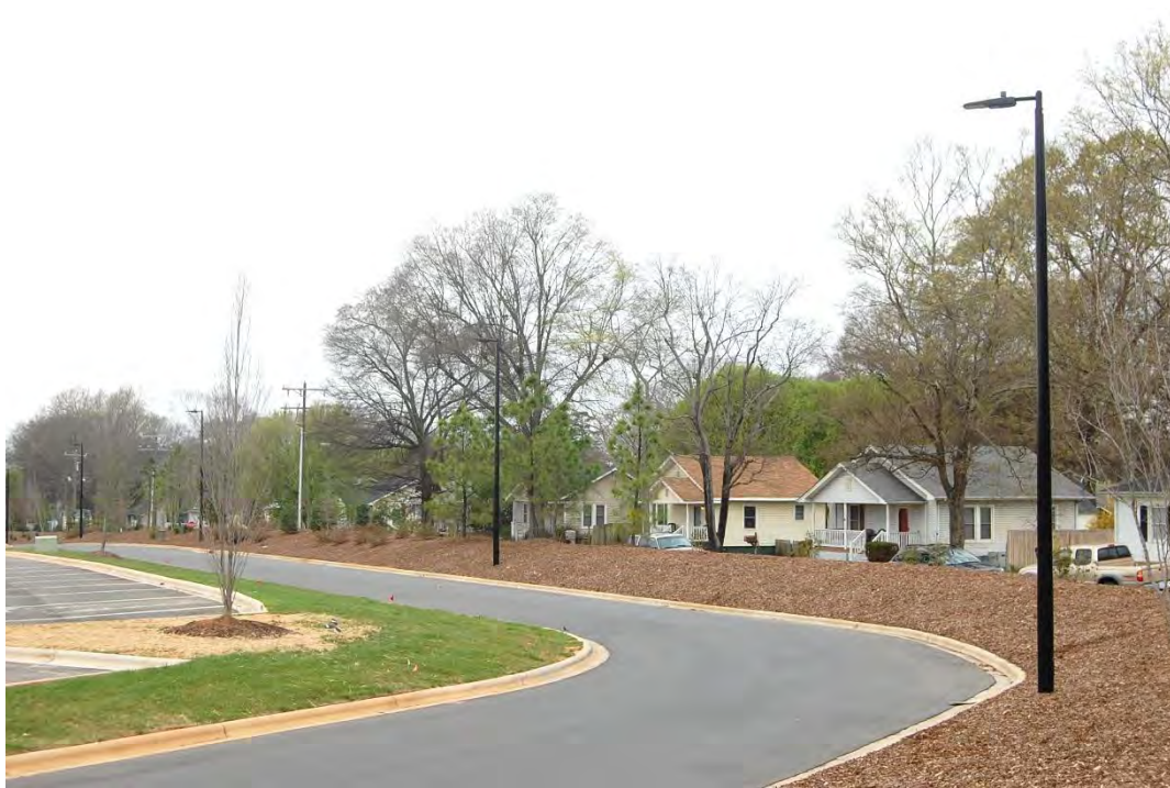
Belmont Fabric Company-South Fork Manufacturing Company Mill Village, Looking Northwest Towards Live Oak Avenue From Modern Parking Lot (Original Mill Site).
