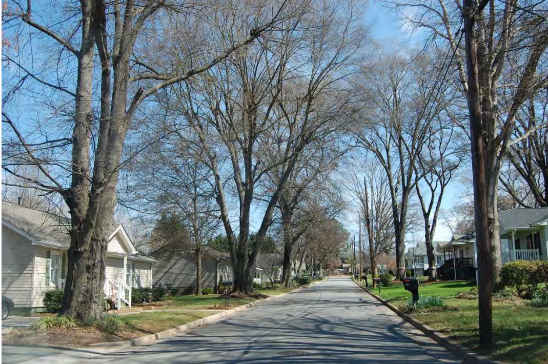
Belmont Fabric Company-South Fork Manufacturing Company Mill Village, Rankin Street, Looking East From Cross Street.
