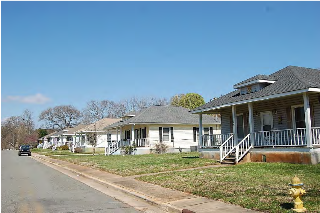
Stowe Spinning Company Mill Village, 1920, Jackson Street, Belmont, Looking North.
